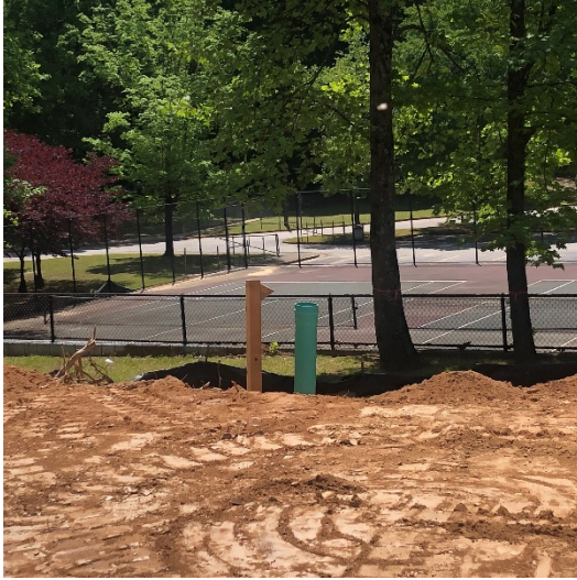
Sanitary Cleanout Install
