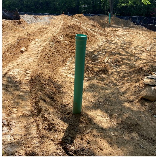
Sanitary Cleanout Install
