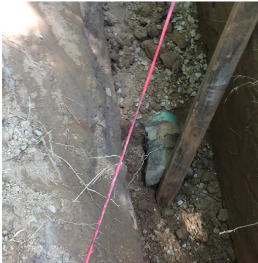
Sanitary Sewer Line Install and Backfill
